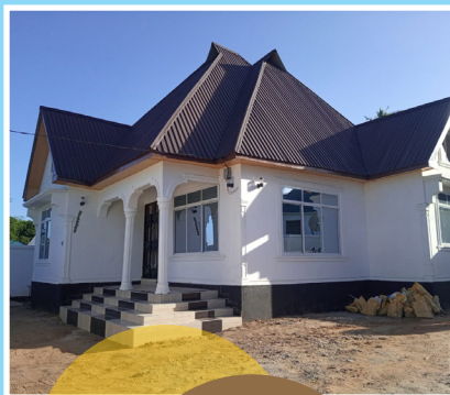
JENGO LA PEKE YAKE (DETACHED BUILDING)
